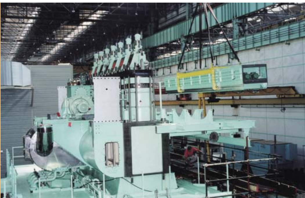
Installing the rail unit.
