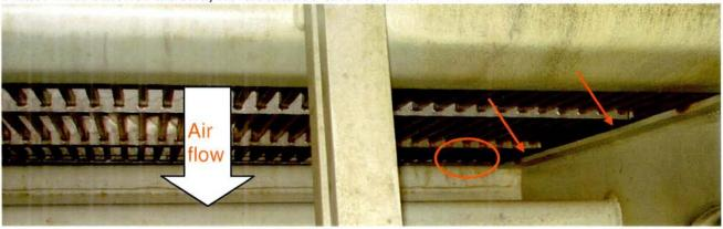
Green arrow = bolt ends are visible Green circle = gap indicates correct mounting
