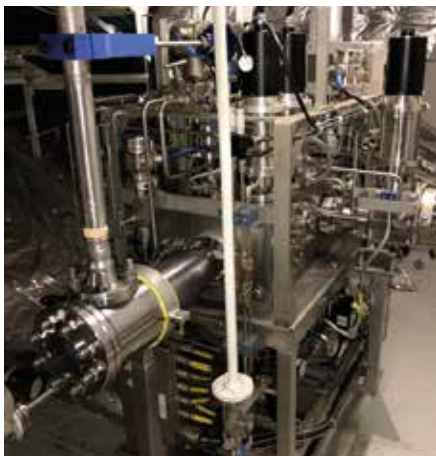
Fig. 17: GVT with inlet filter and slow-opening valve
