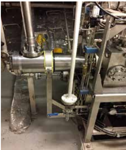
Fig. 20: 10 micron fine filter before the GVT
