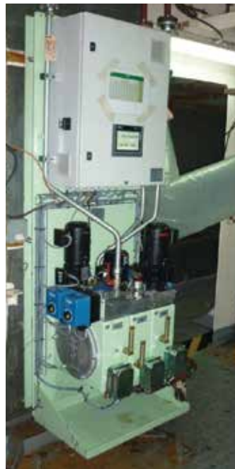
Fig. 9: Automated cylinder oil mixing (ACOM) unit
