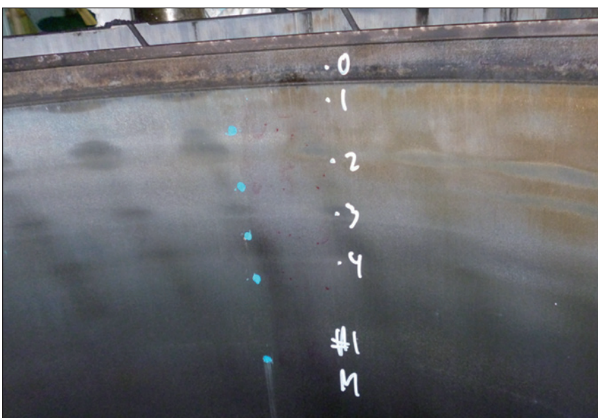
Fig. 26: Cold corrosion in the top of the cylinder liner
