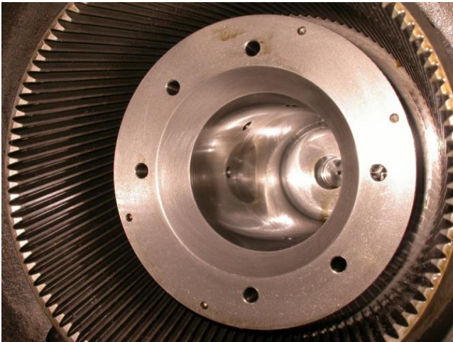
Figure 16: Photograph of the outer helix gear inside the valvedrive after 31,882 hours.
