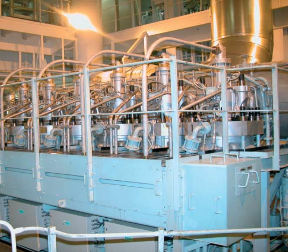
Rail unit at the cylinder top level of the 6RT-flex50 engine, with the electronic control units on the front for good access.
